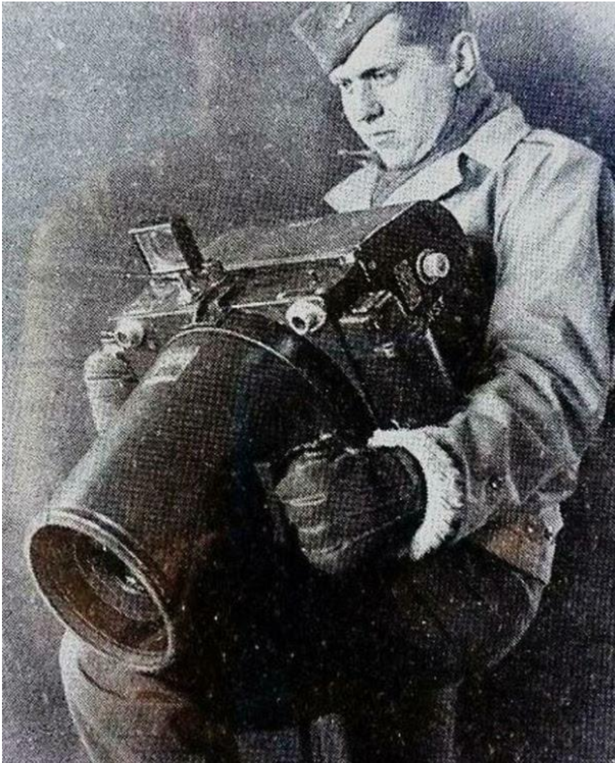
7 - Kodak K-24 camera, used for aerial photography during WW2 by the Americans.
